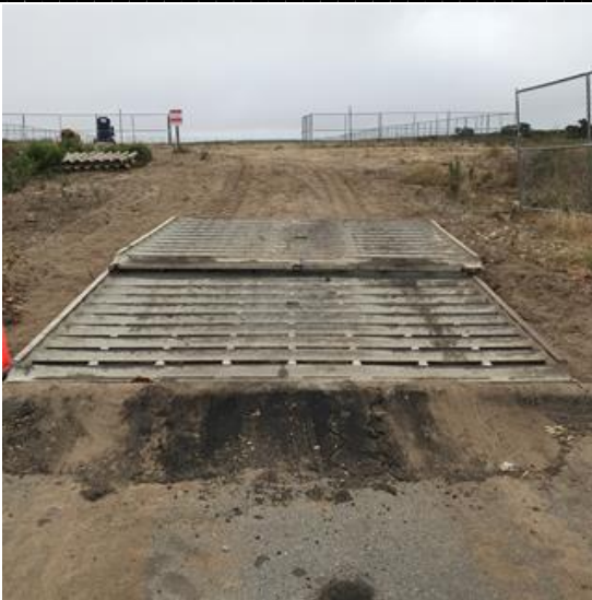
Begin work on staging area entrance
